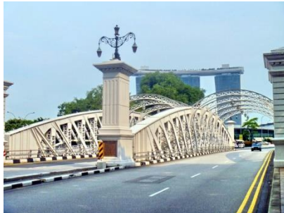
B2. Anderson Bridge
