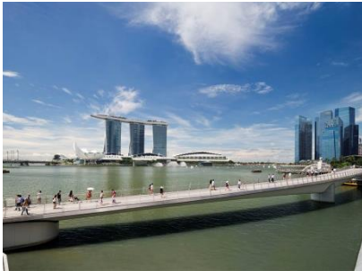
B1. Jubilee Bridge
